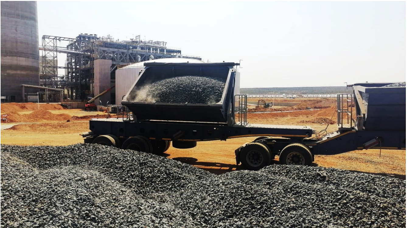
Material handling and transport at a project site
